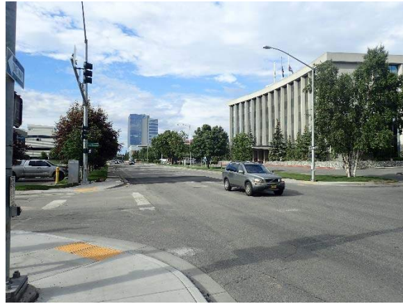
Photo 28 - Intersection Sight Distance Obstructions (W. 32 nd Ave. & C St.)
