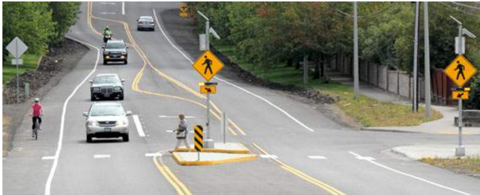
Photo 33 - Midblock Crossing with Pedestrian RRFB ( http://www.co.washington.or.us/LUT/TrafficSafety/DrivingSafety/rrfb.cfm )
