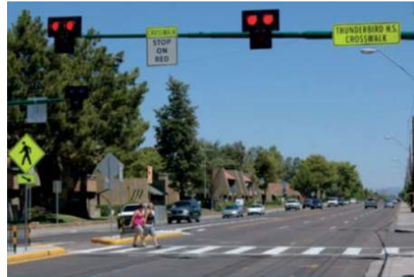
Photo 31 - Pedestrian Hybrid Beacon ( https://safety.fhwa.dot.gov )
