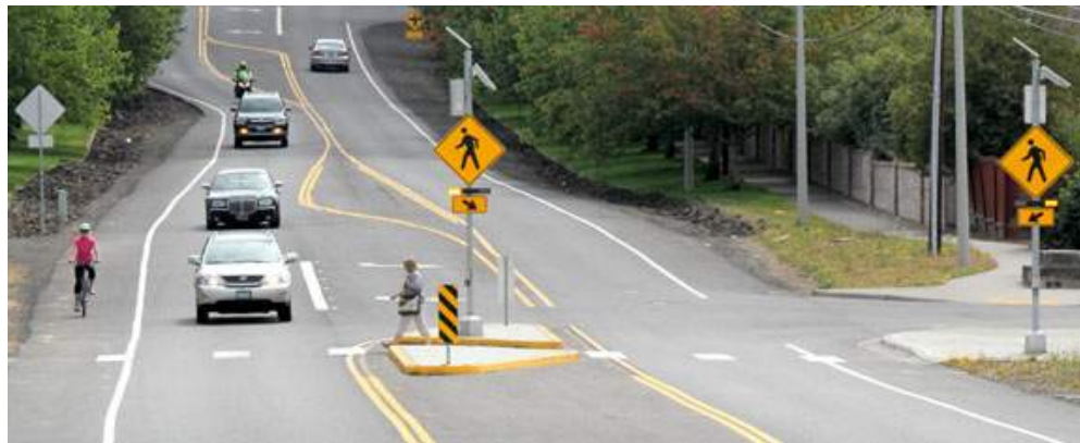
Photo 30 - Midblock Crossing with Pedestrian RRFB ( http://www.co.washington.or.us/LUT/TrafficSafety/DrivingSafety/rrfb.cfm )
