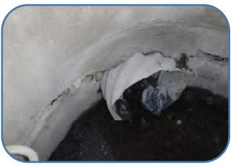
effluent cracked around pipe connections
