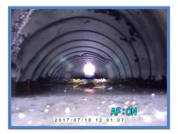
6-inches of debris in invert blocking flow
