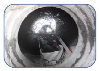
12-inch effluent and cracked grout
