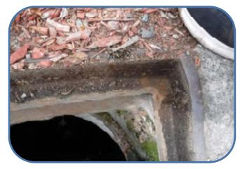
MH frame corrosion on frame
