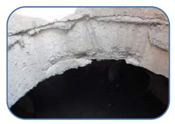
reinforcement exposed in reducing slab
