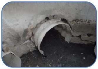
effluent with crack between pipe connections
