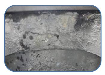
crack in reducing slab not seperated
