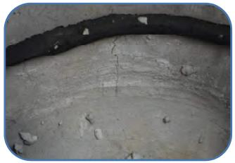
small crack in base above effluent pipe
