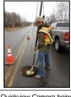
Quickview Camera-being lowered into pipe
