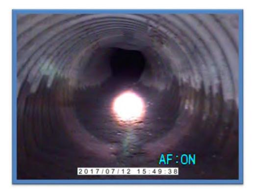
Photo 1-Dent in crown of pipe between 11 o'clock and 1 o'clock
