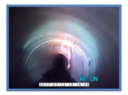
Photo 1-root intrusion at crown
