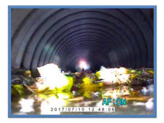
Photo 1-6 inches of debris in invert blocking flow
