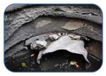
12-inch effluent cracked grout
