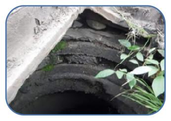
cracked chimney with hole
