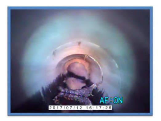
Photo 2-root intrusion at 4 o'clock
