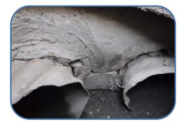
pipe 5-effluent and pipe 4- influent cracked base
