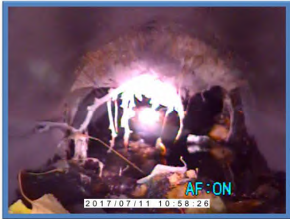
Photo 1-Hole in crown of pipe between 10 o'clock and 2 o'clock position
