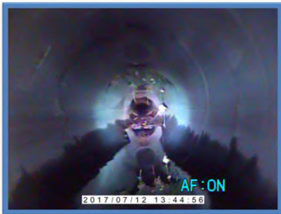
Photo 5-Hole in pipe at 10 o'clock position
