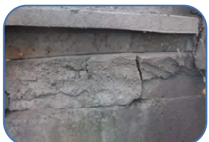
cracked and broken chimney
