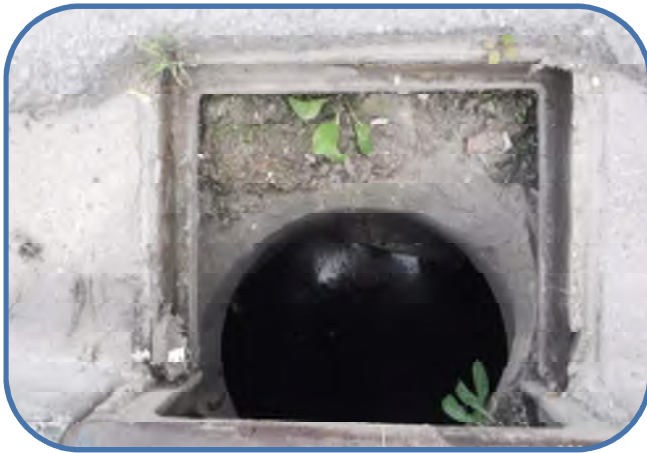
Offset frame from manhole
