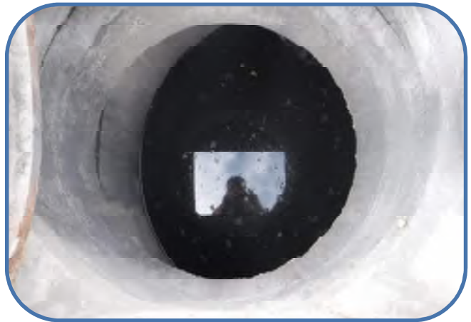
chimney and reducing slab
