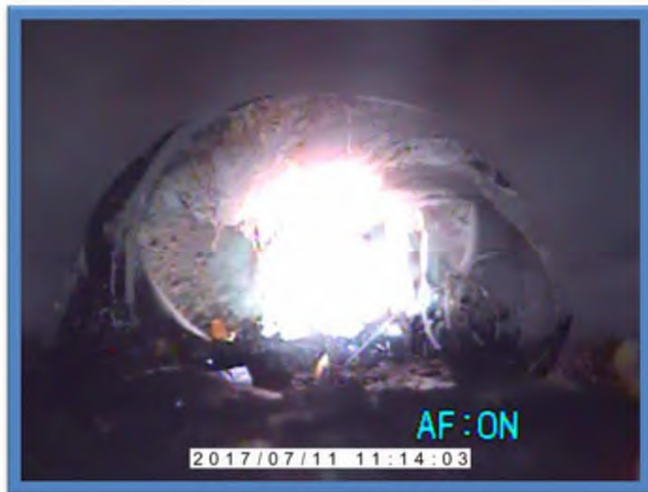
Photo 2-Pipe collapsing between 7 and 11 o'clock soil void visible behind hole.
