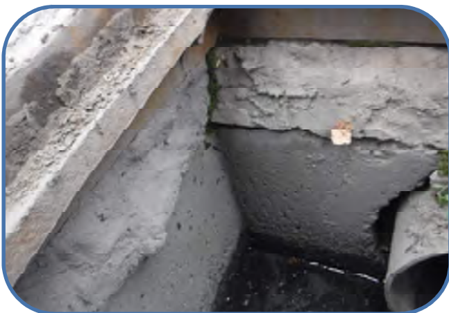
grout cracked on chimney
