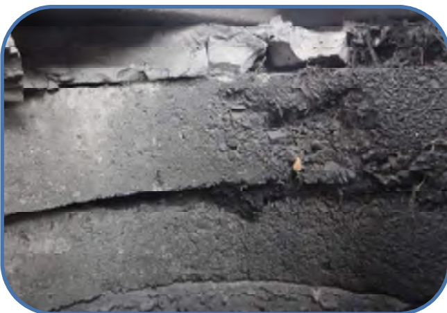
grout cracked between frame and chimney
