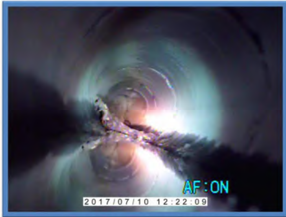
Photo 1-Possible hole in pipe at 8 o'clock with root intrusion.
