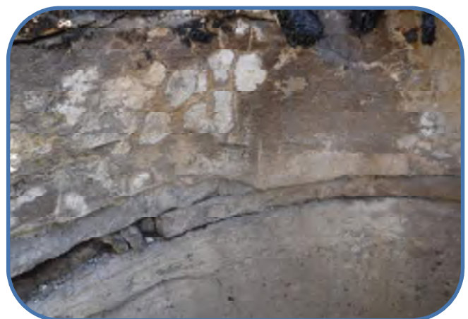
grout cracked
