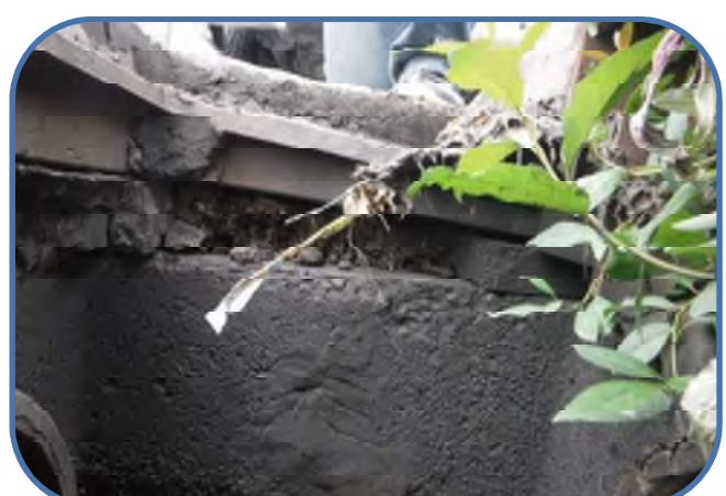
grout cracked in chimney
