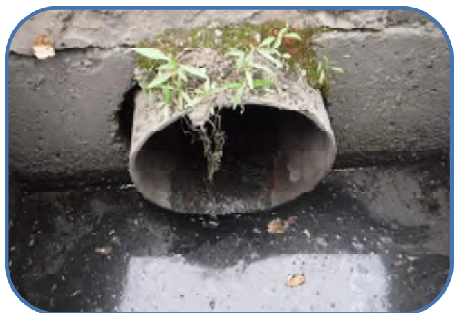
base and pipe penetration. no grout
