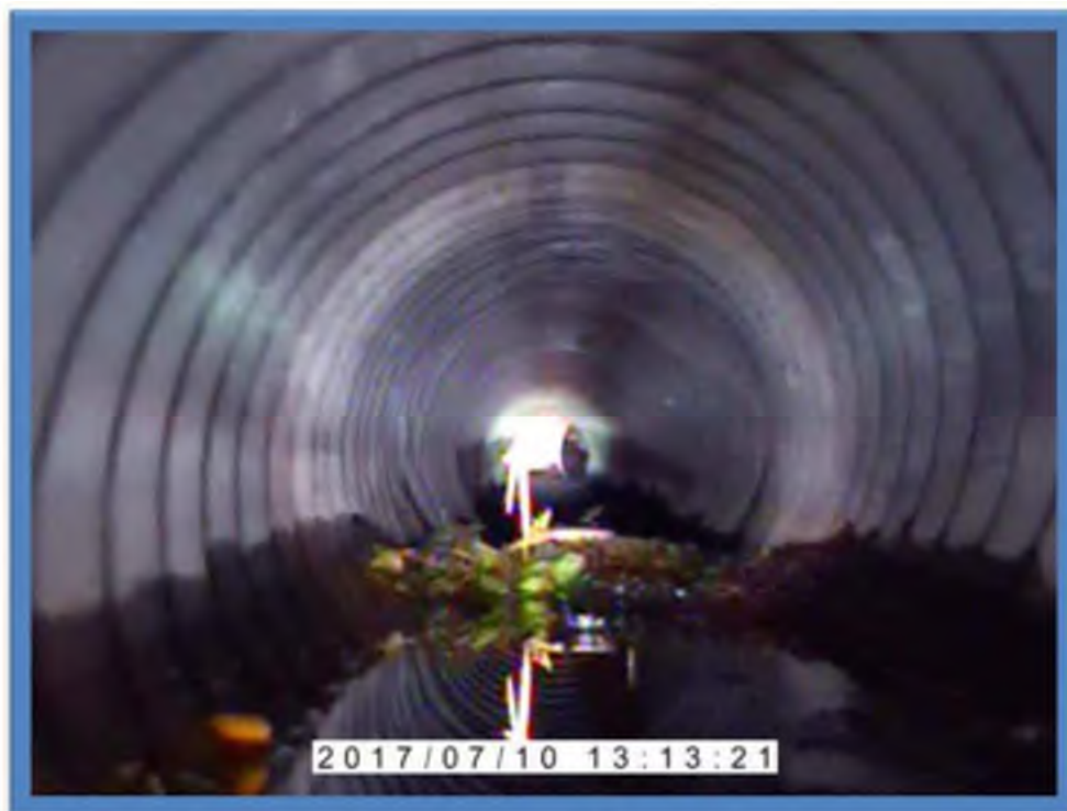
Photo 1-4 inches of debris in invert blocking flow
