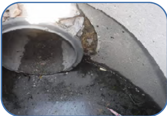
effluent missing grout
