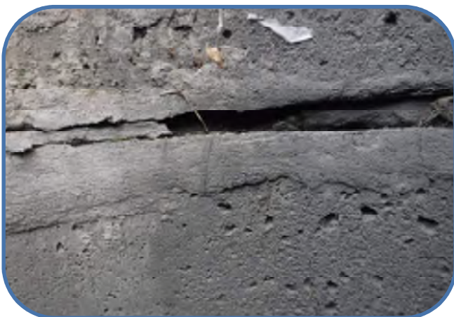
grout cracked between risers
