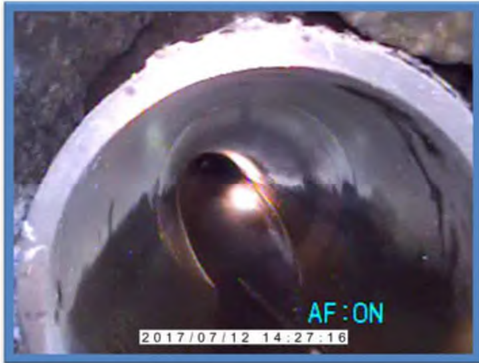
Photo 1-Standing water in pipe
