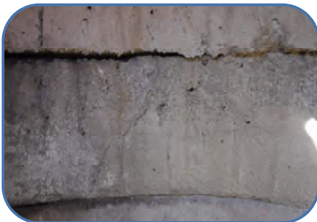
influent with cracked grout
