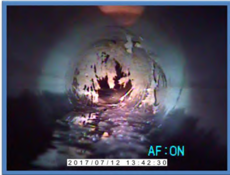
Photo 2-Holes in pipe and root intrusion
