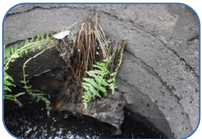
vegetation growing between chimneys and reducing slab
