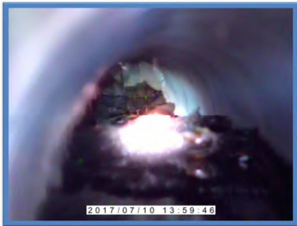
Photo 1-5 inches of debris in invert blocking flow
