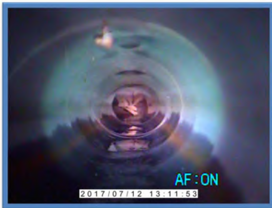
Photo 1-Ovality in pipe section near manhole 1631-132
