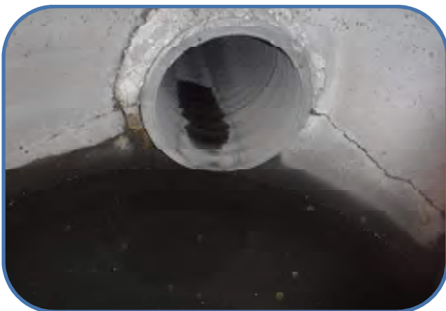
influent 12-inch pipe cracked
