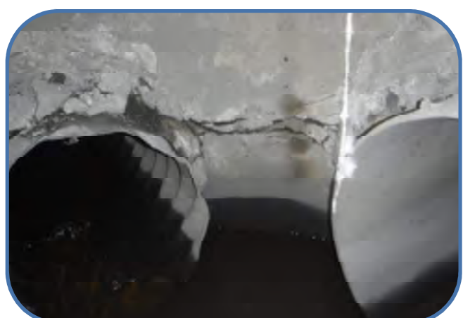
effluent pipe and crack in base
