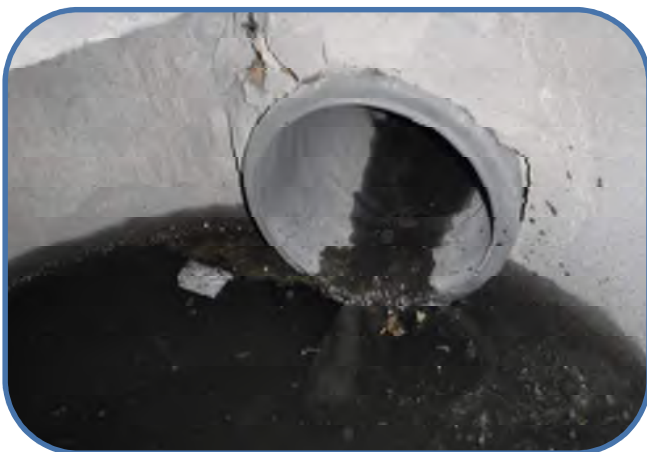
grout cracked on effluent pipe
