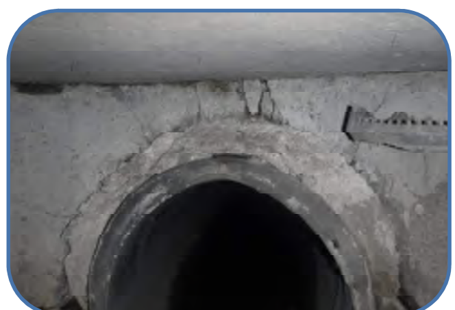
effluent 18-inch pipe cracked
