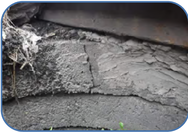
cracked chimney
