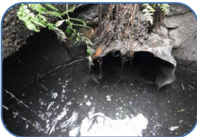
12-inch effluent cracked grout
