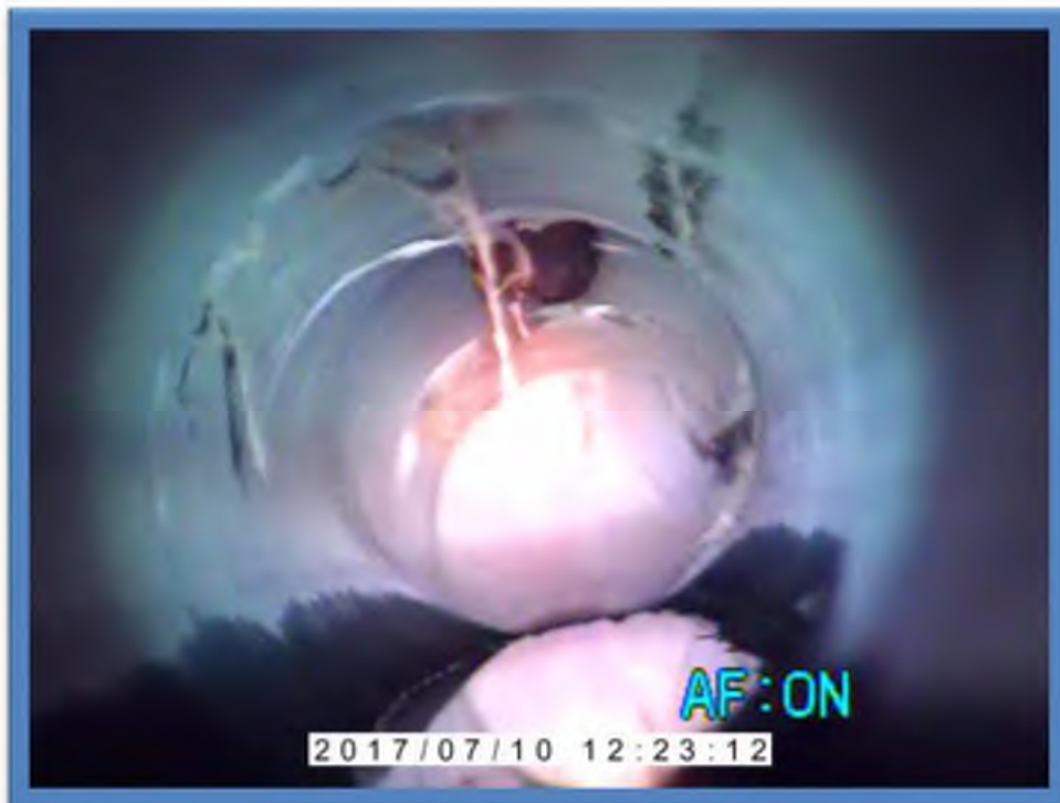
Photo 2-Root intrusion at joint within pipe.
