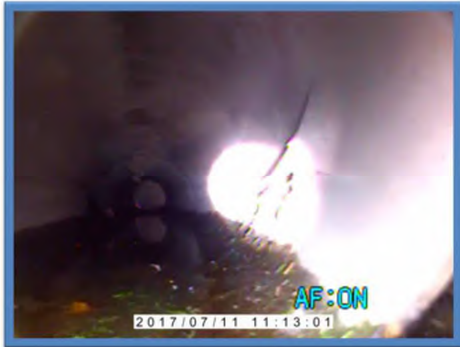
Photo 1-Hole in pipe at 5 o'clock position
