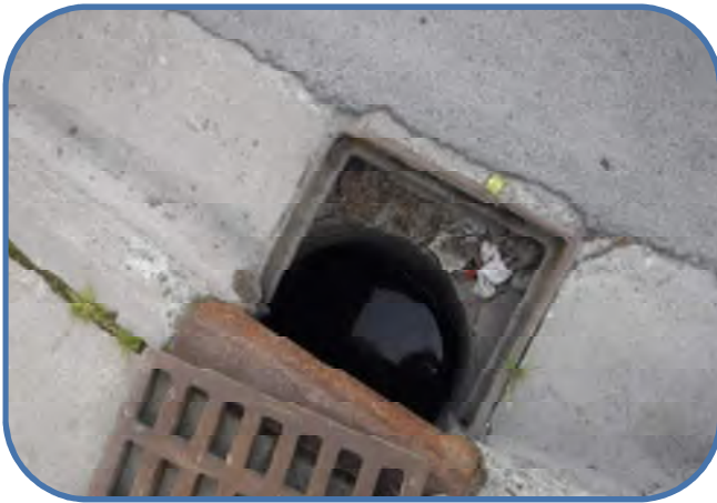
offset frame from riser
