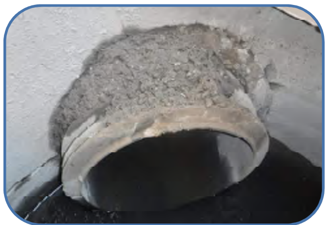
18-inch influent grout missing soil visible
