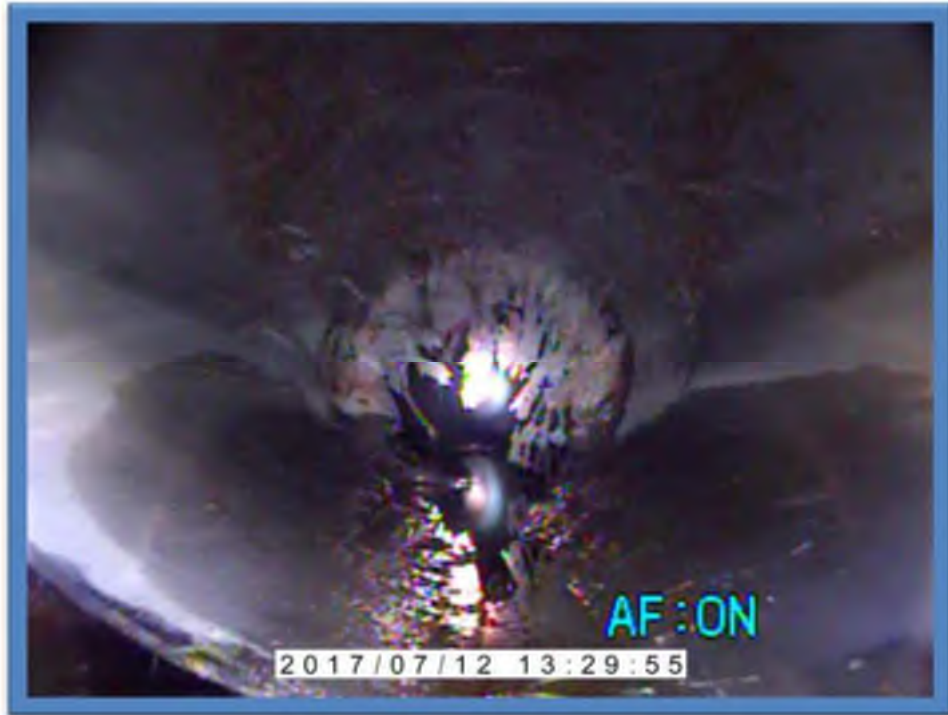
Photo 1-Root intrusion in pipe
