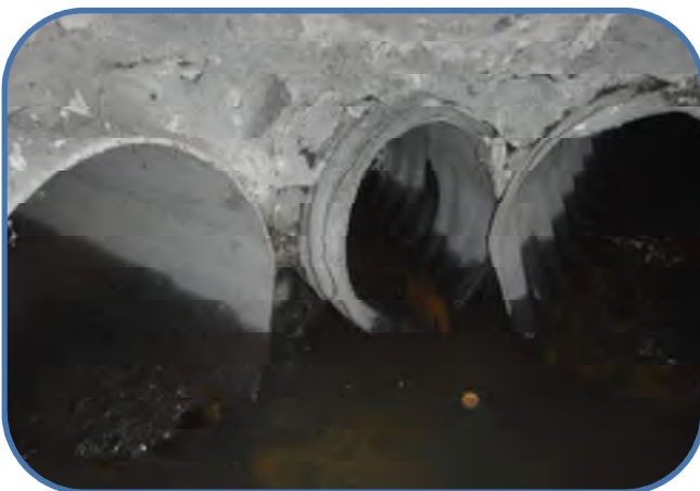
influent pipes, 12-inch CPEP could not find end on surface or with quickview
